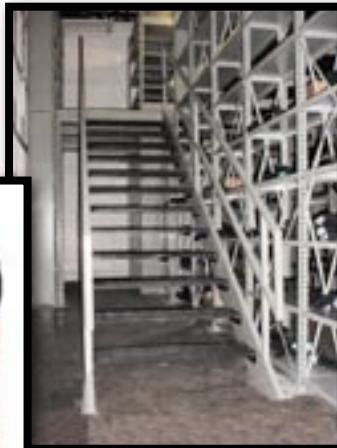
CUSTOM STAIRS & PLATFORMS
